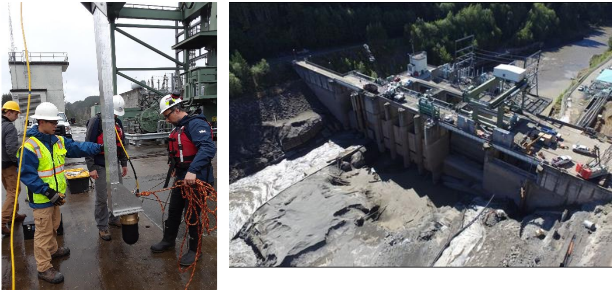
Figure 1. Images showing the DAS deployment at the Cowlitz Hydroelectric facility.
