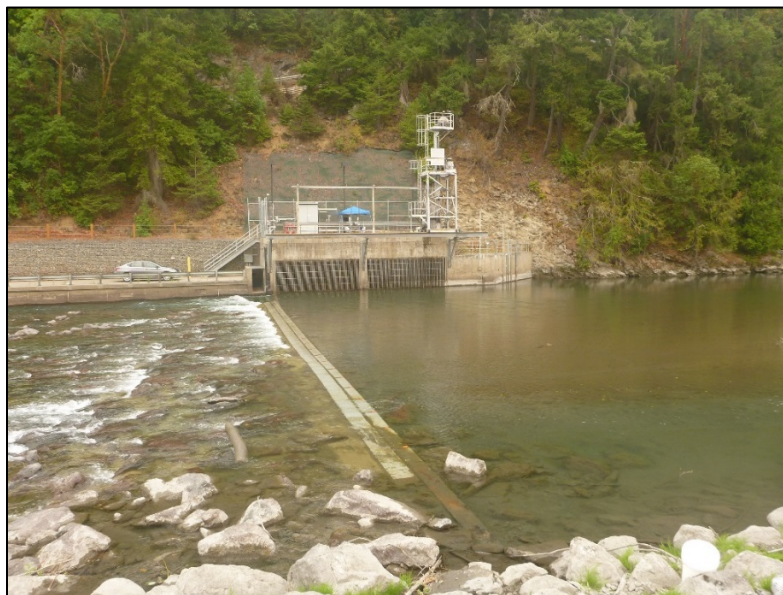
Figure 2. Photograph of the concrete weir and impact plate system mounted to the downstream side. The intake structure is in the background. Flow (approximately 11.3 \text{ m}^3/\text{s} ) is from right to left in the photograph (Sep. 2017).
