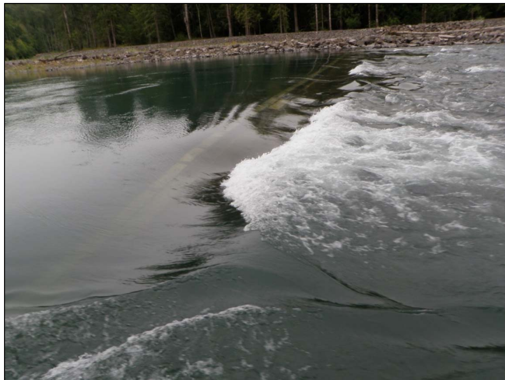
Figure 4. Pre-dam-removal view from the ESWI structure looking across the weir in July 2010. Flow is left to right, 28.3 cms. The plates can be seen beneath the hydraulic jump at the crest of the riffle.
