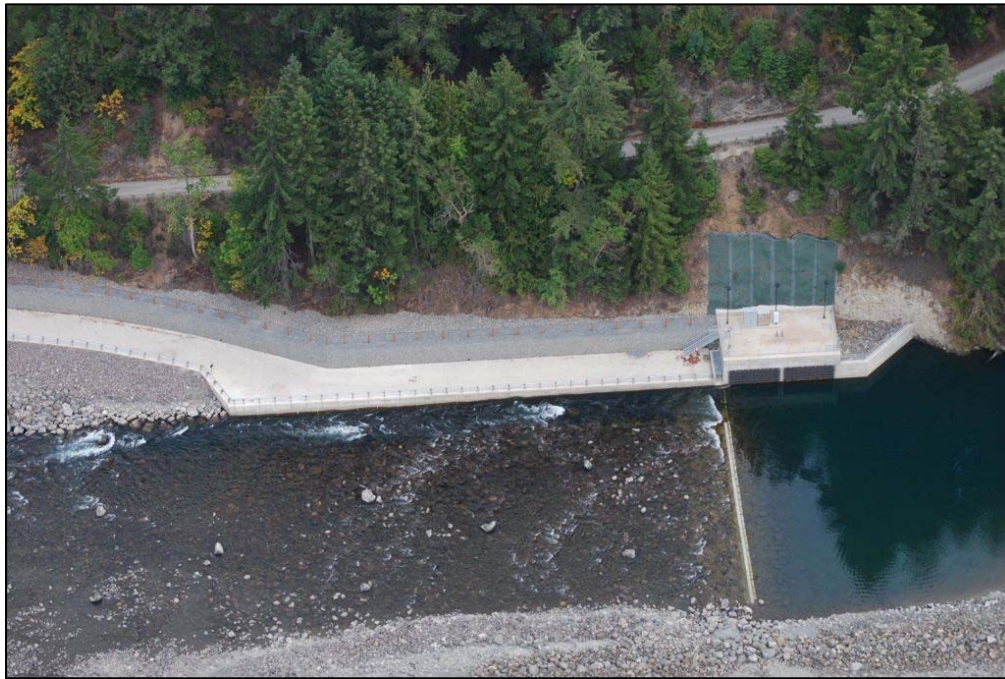
Figure 3. Aerial view of the weir at ESWI (2008) after installation. Flow is from right to left. Low flow notch is evident along the margin of the concrete structure (photo courtesy Andy Ritchie, USGS).
