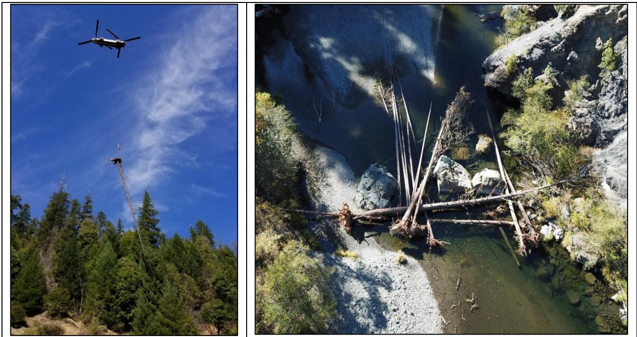
Figure 2. Example Photos showing Chinook Helicopter Flight and Large Wood Geomorphic Structure Placement
