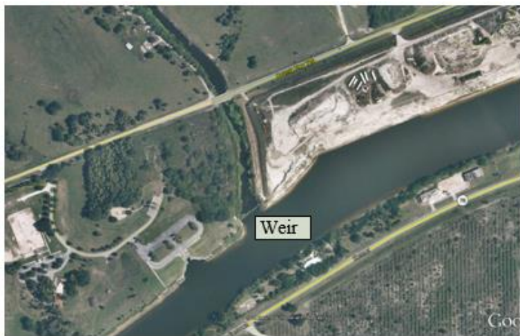
Figure 6. Lateral inflow structure discharging into the C-44 canal, near the C-44 reservoir
