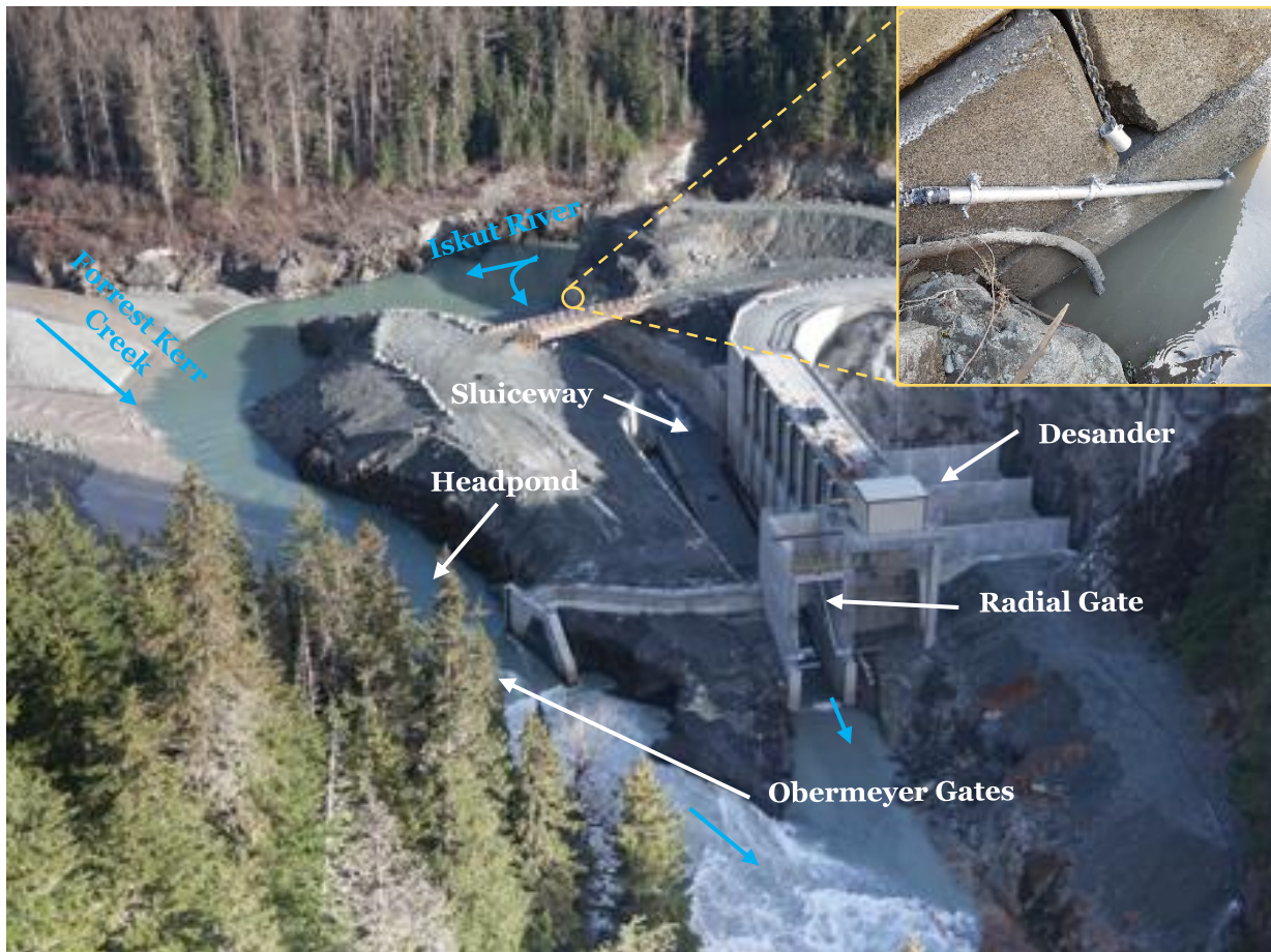
Figure 2. Aerial view of the Forrest Kerr hydropower facility and location of the hydrophone sensor (image from Bethany Duarte, HydroReview)
