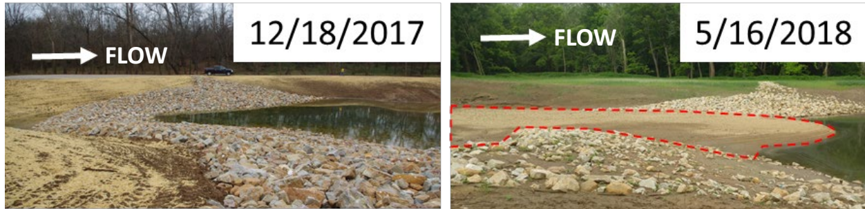
Figure 5. Deposition of coarse sediment at the upstream entrance to trap; during low water (Pics: J.Collum)
