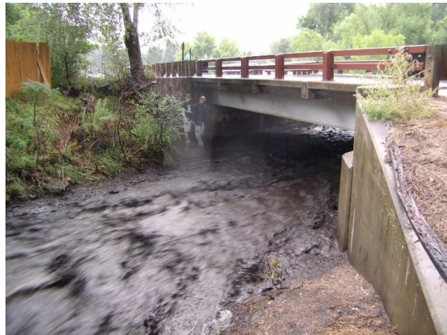
Figure 4. High flows generated by a summer thunderstorm with high concentrations of suspended sediment and ash at the outlet of the 14 km 2 Hill Gulch watershed in summer 2012, two months after the High Park Fire.
