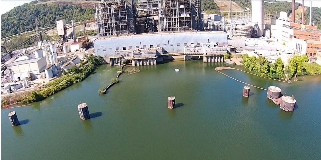
Figure 1. Aerial view of the Cardinal Plant forebay (IIHR, September 21, 2015)
