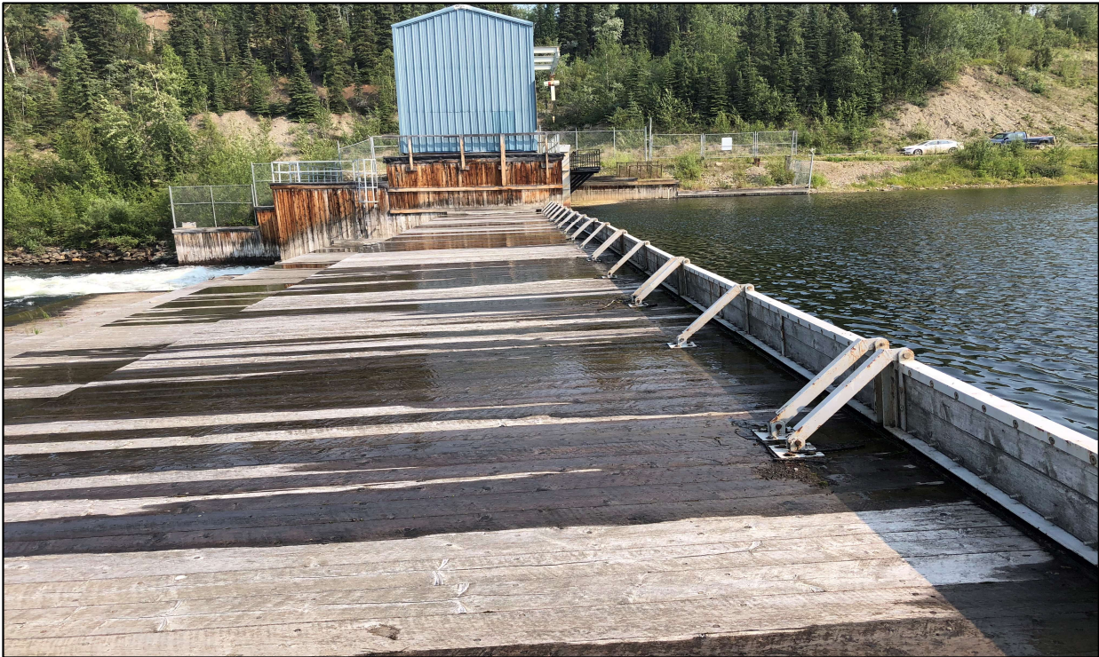
Figure 8. Mayo Lake Control Structure
