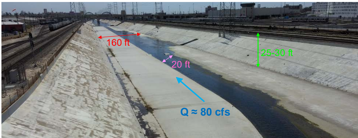
Figure 1. Los Angeles River looking downstream from 1 st Street, annotated with approximate dimensions and base flow rate
