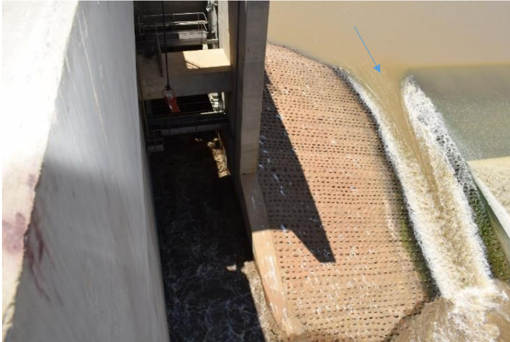
Figure 6. Eelway viewed from downstream
