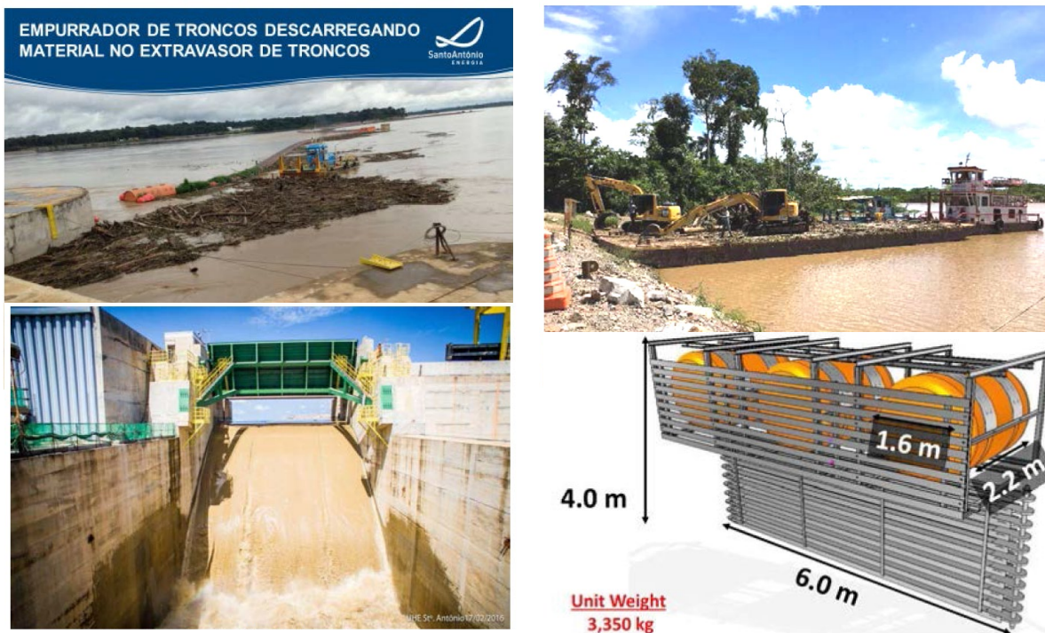
Figure 2. Examples of equipment and methods used to prevent debris and LW from damaging hydroelectric facilities at Santo Antônio dam. Upper left: “Wood pusher” tug boat, log boom, and log chute. Upper right: Tug, barge and excavators to remove logs that get through/under/around booms. Lower left: log chute spillway; lower right: typical floating log boom unit in reservoir
