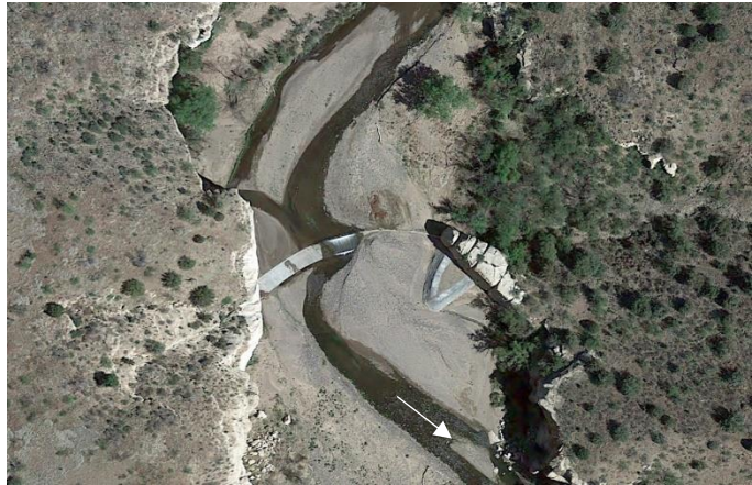
Figure 1. Blue River Fish Barrier (4/13/2014). The depositional bar that formed on river left has buried the structure apron.
