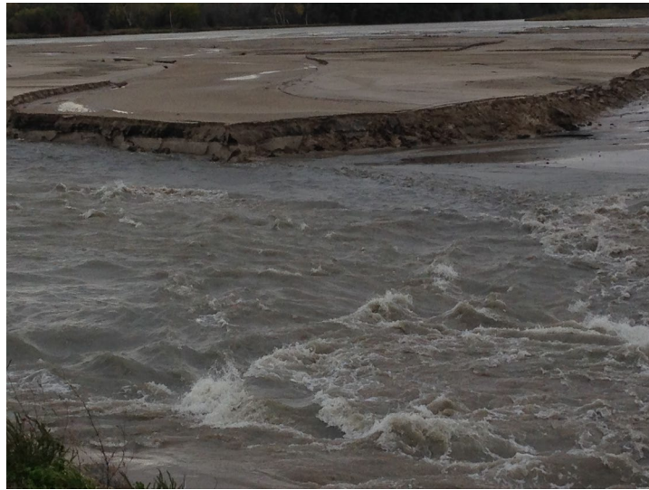
Figure 2. Photograph of the Spencer Dam reservoir during the October 2014 sediment flush looking upstream from right bank. The streamflow is moving towards the bottom right corner.
