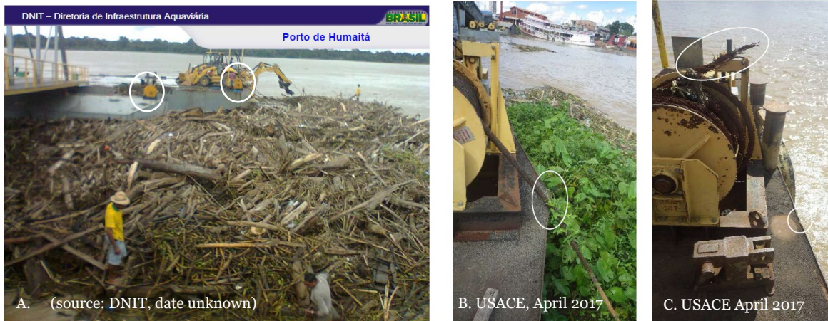
Figure 3. A. Major debris accumulation at Humaitá IP-4 port; B. Porto Velho IP-4 port facility damage: Mooring winch upstream side, with frayed cable under load; C. failed mooring winch cable, and damaged barge, downstream side
