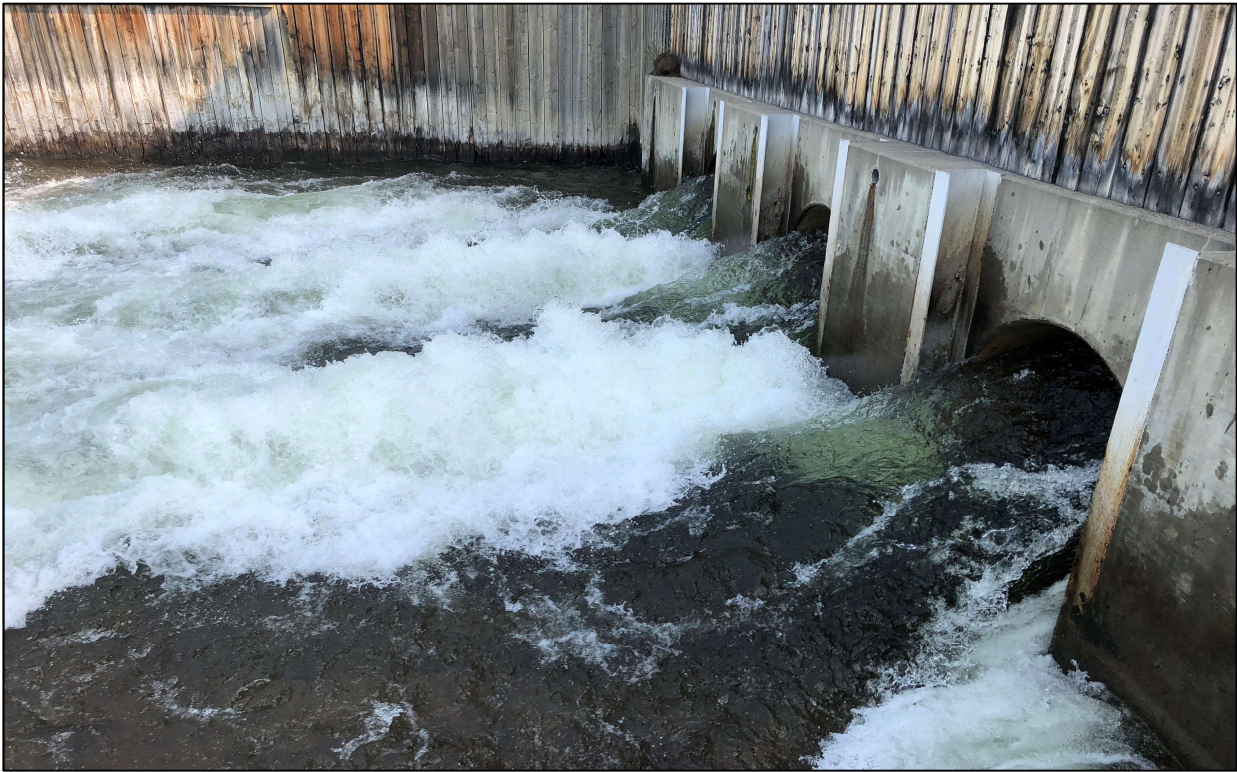
Figure 9. Mayo Lake Control Structure bottom outlets
