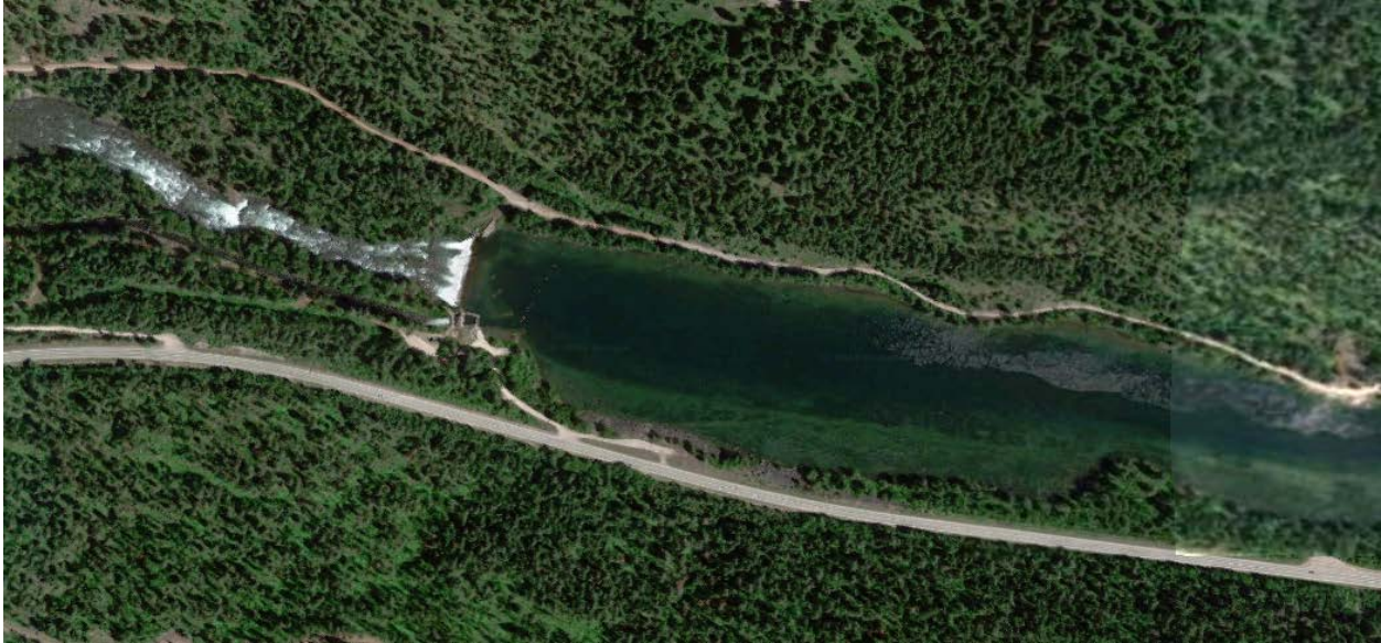
Figure 3. Aerial photo of the Montana hydroelectric project
