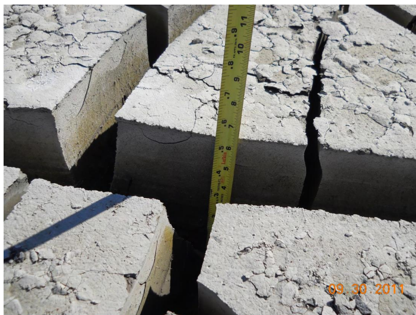
Figure 1. Clay fissures in dry watershed conditions (West Consultants, 2012)
