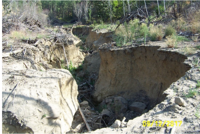
Figure 1b. Close up showing gully incision in Brender Creek (previous figure), 2017. Up to 7 m (21 ft) of downcutting happened in 2017, shortly after the site was logged (Figure 1a). Photo courtesy of Washington Department of Fish and Wildlife and Chelan County Natural Resources.
