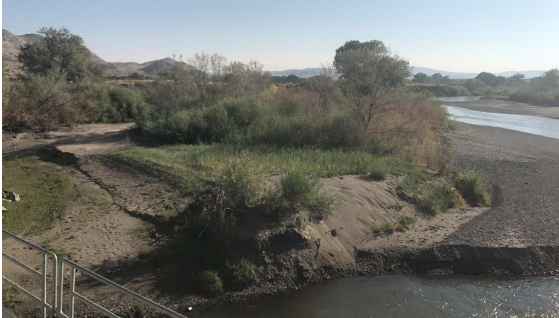
Figure 10. Upstream view of reservoir sedimentation following 2017 flood in vicinity of fish passage release and radial gate.
