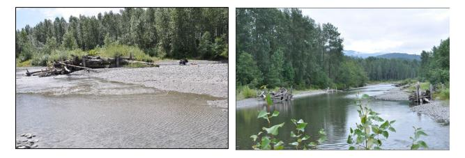
Photos show ELJ in the study reach. The photo on the left is a ELJ at the head of a gravel bar. Note the people on the bar for scale. The photo on the right is looking upstream at a reach where ELJ were constructed on opposite banks.
