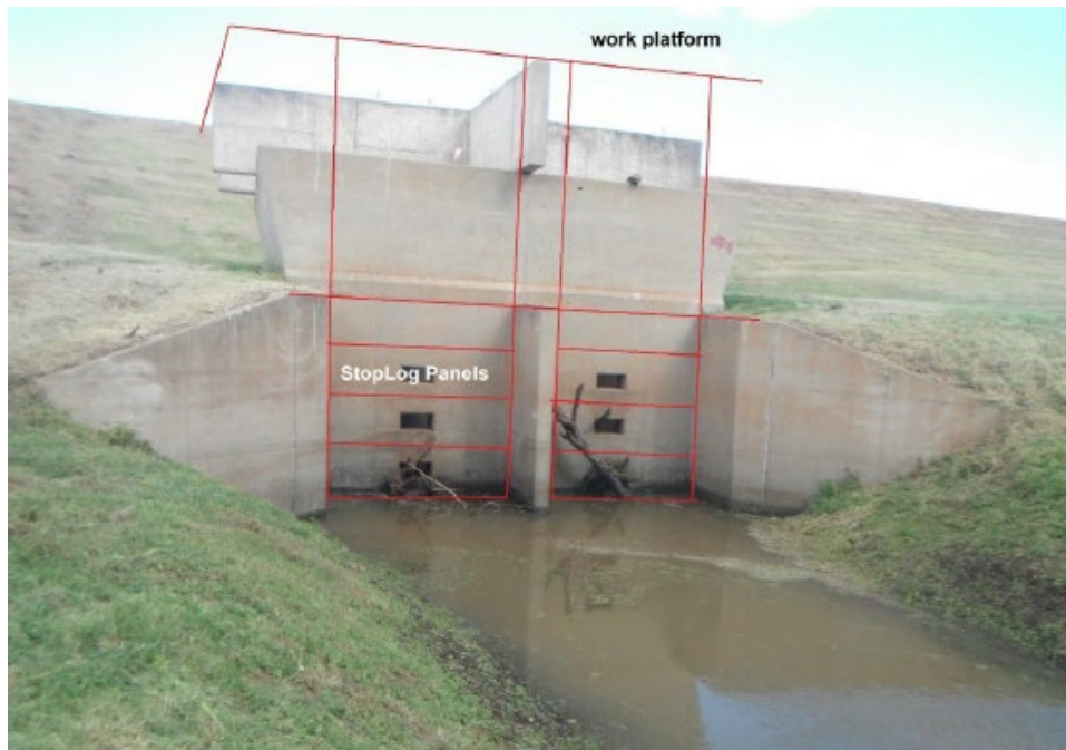
Figure 9. Proposed StopLog Panels and Work Platform at the Honokōwai Dam riser structure
