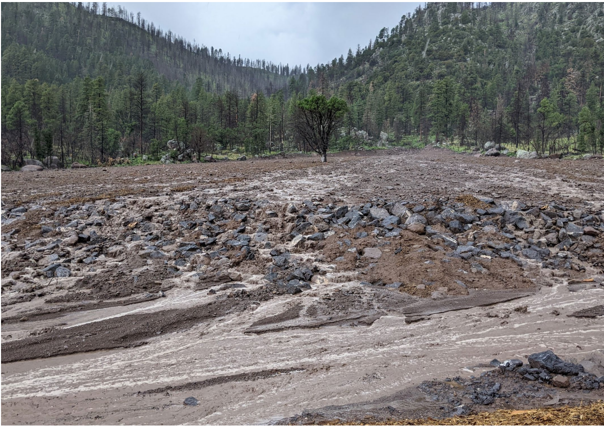
Figure 9. Ginger alluvial fan work site (looking upstream) during a 2022 flow event, note the spread of flow and subsequent drop in water velocity allowing sediment aggradation.
