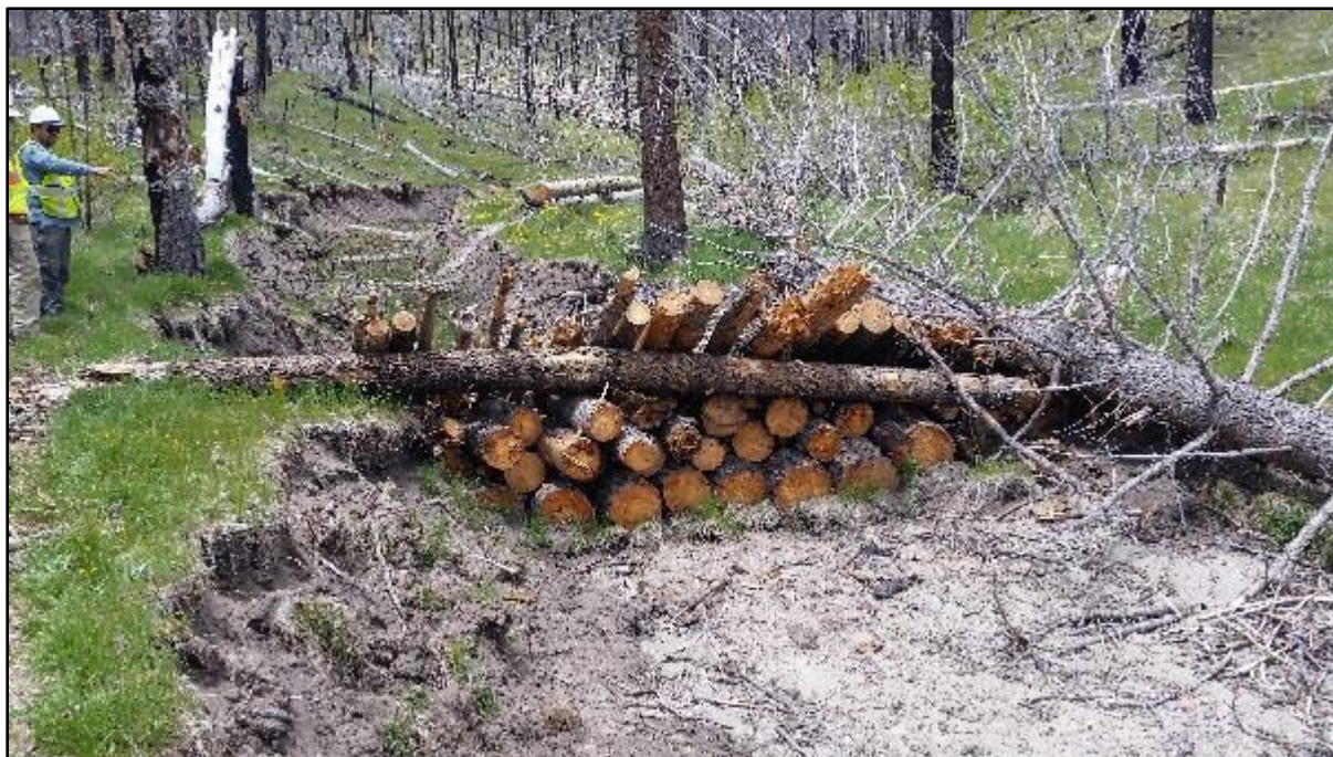
Figure 8. Erosion Control Structures in New Mexico.
