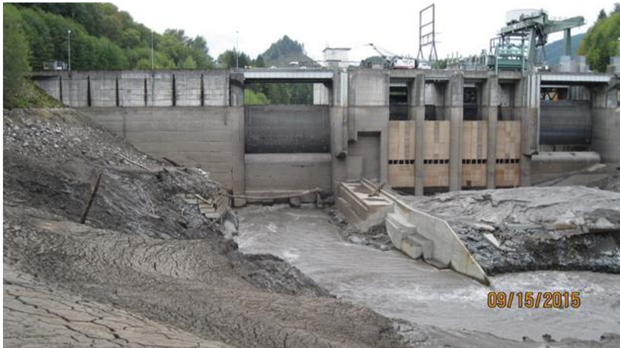
Figure 4. Photo of the hydroelectric structure during drawdown illustrating many of the same structures that the scan shows.
