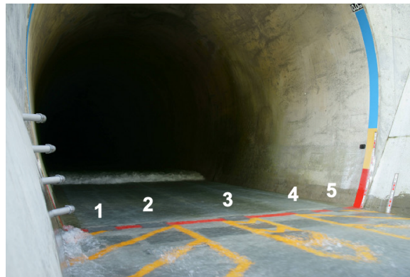
Figure 2. Koshiibu SBT outlet part with five IPs for bedload monitoring
