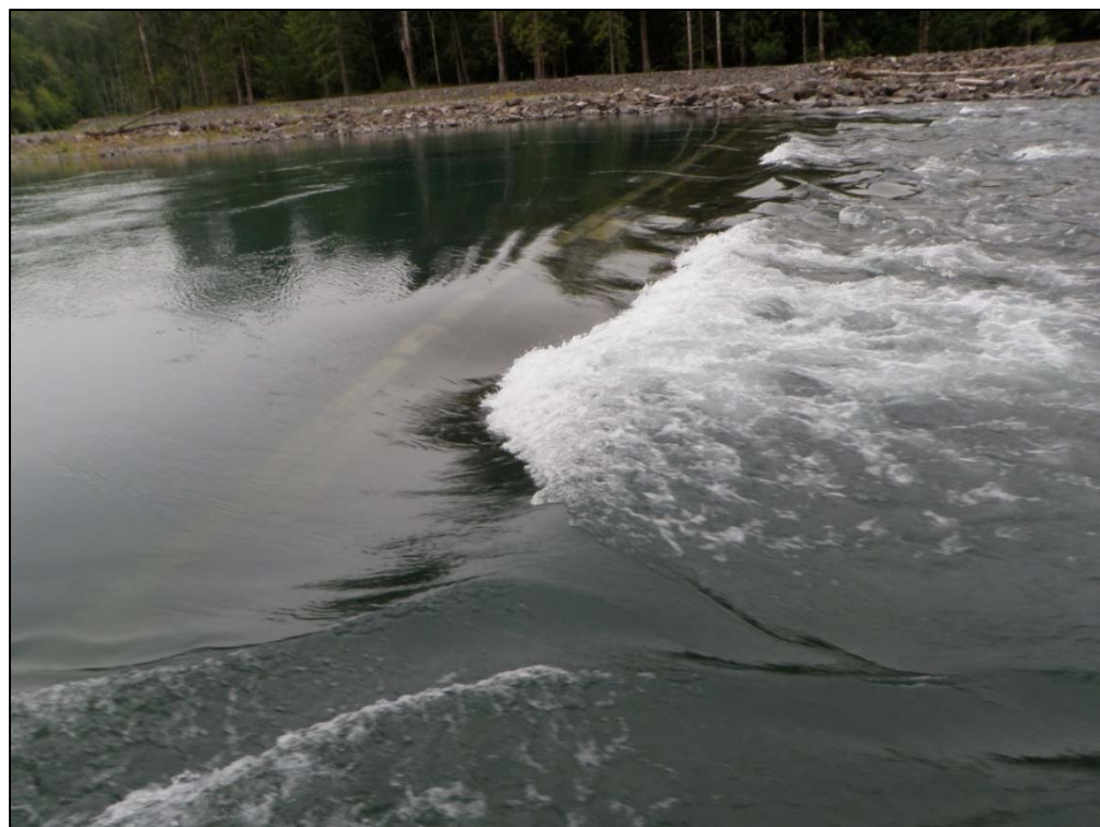
Figure 4. Pre-dam-removal view from the ESWI structure looking across the weir in July 2010. Flow is left to right, 28.3 cms. The plates can be seen beneath the hydraulic jump at the crest of the riffle.
