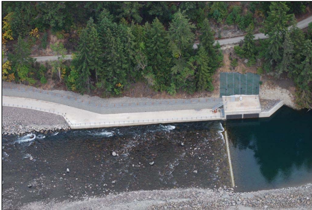
Figure 3. Aerial view of the weir at ESWI (2008) after installation. Flow is from right to left. Low flow notch is evident along the margin of the concrete structure (photo courtesy Andy Ritchie, USGS).
