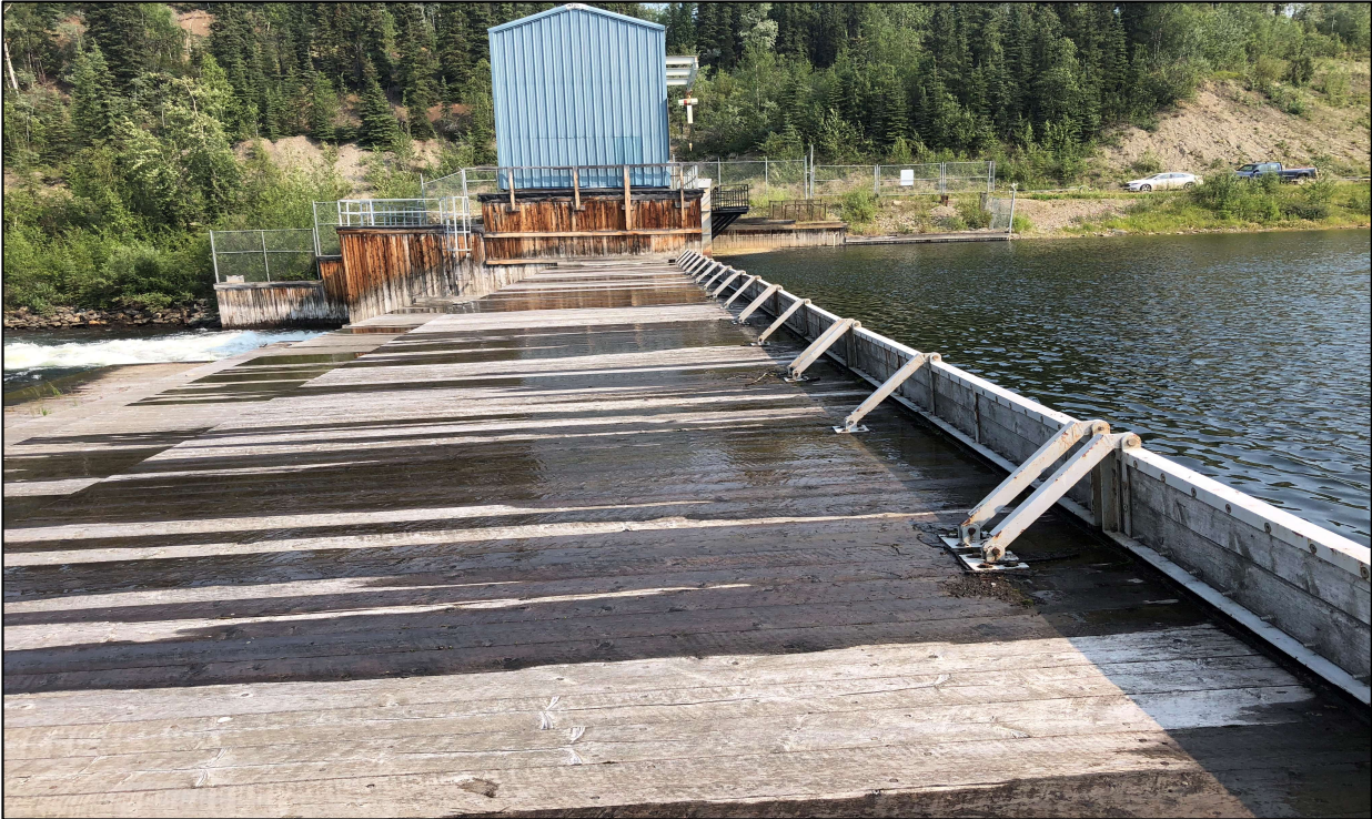
Figure 8. Mayo Lake Control Structure
