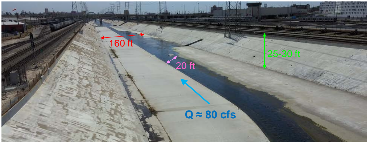
Figure 1. Los Angeles River looking downstream from 1 st Street, annotated with approximate dimensions and base flow rate
