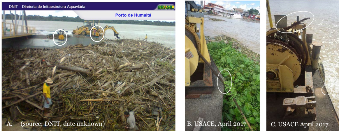
Figure 3. A. Major debris accumulation at Humaitá IP-4 port; B. Porto Velho IP-4 port facility damage: Mooring winch upstream side, with frayed cable under load; C. failed mooring winch cable, and damaged barge, downstream side
