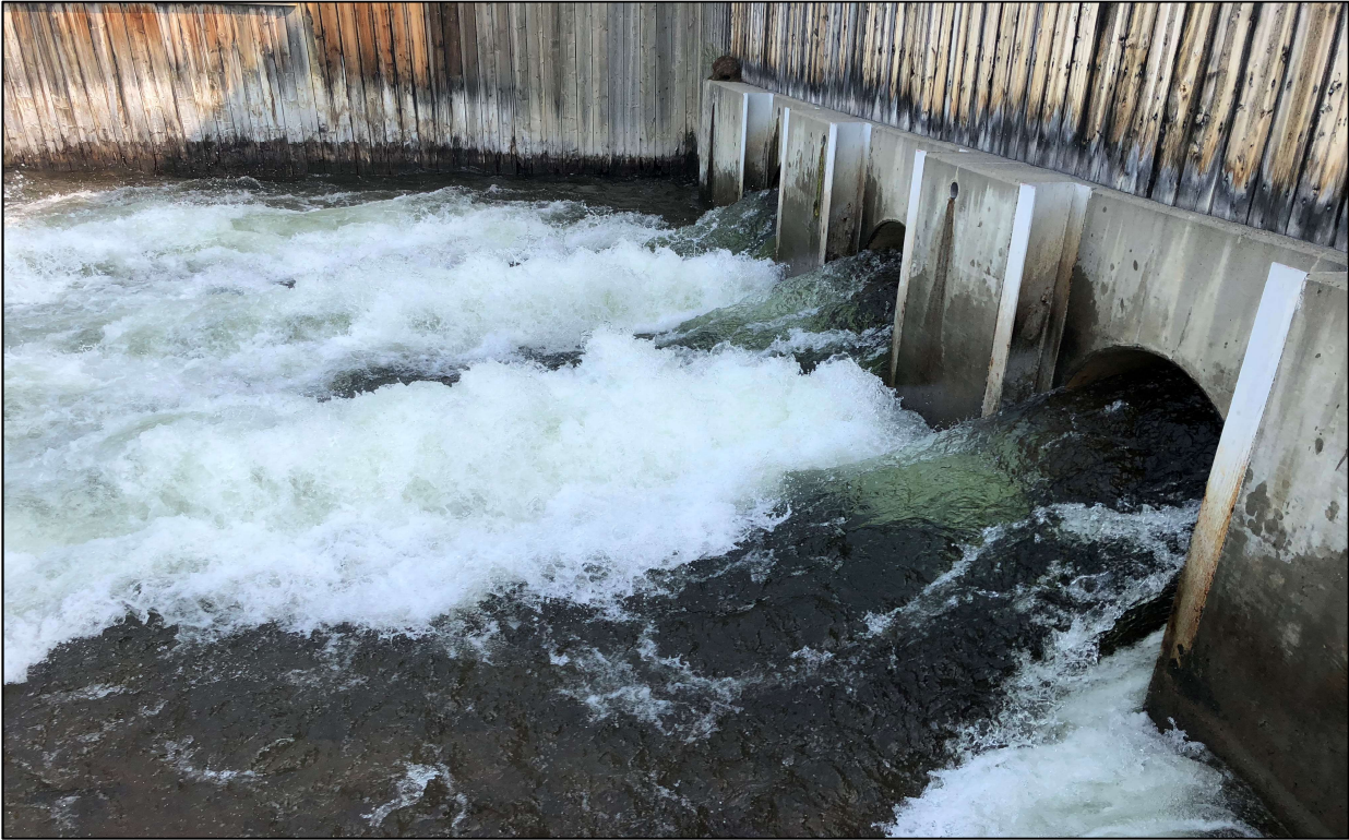
Figure 9. Mayo Lake Control Structure bottom outlets
