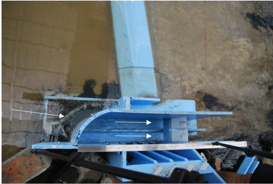
Figure 11. Flushing of the gravel trap at a river discharge of 300 \text{ m}^3/\text{s}
