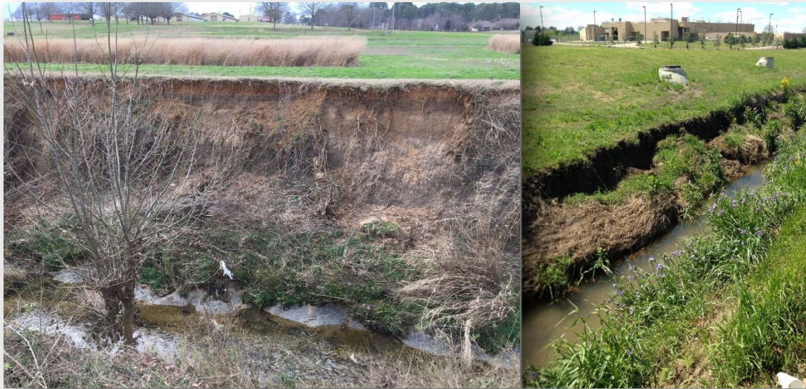
Figure 8. Streambank erosion along main stream and tributaries in the Catalpa Creek watershed
