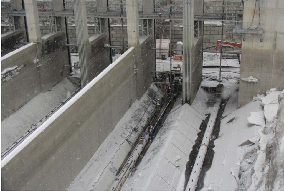
**Figure 3. Air purge system being installed along desander sediment collection pipes. Each slot in the larger pipe is equipped with an air nozzle that blasts material off the sediment collector pipe.**
