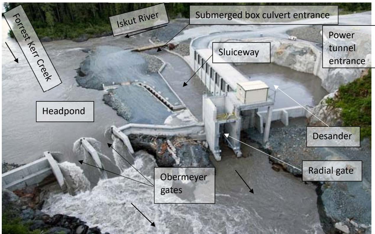
**Figure 1. Aerial view of Forrest Kerr run-of-river facility (box culvert on the bottom of the sluiceway is fully submerged and not visible).**
