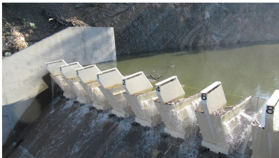
Figure 2. McClure Spillway Fusegates
