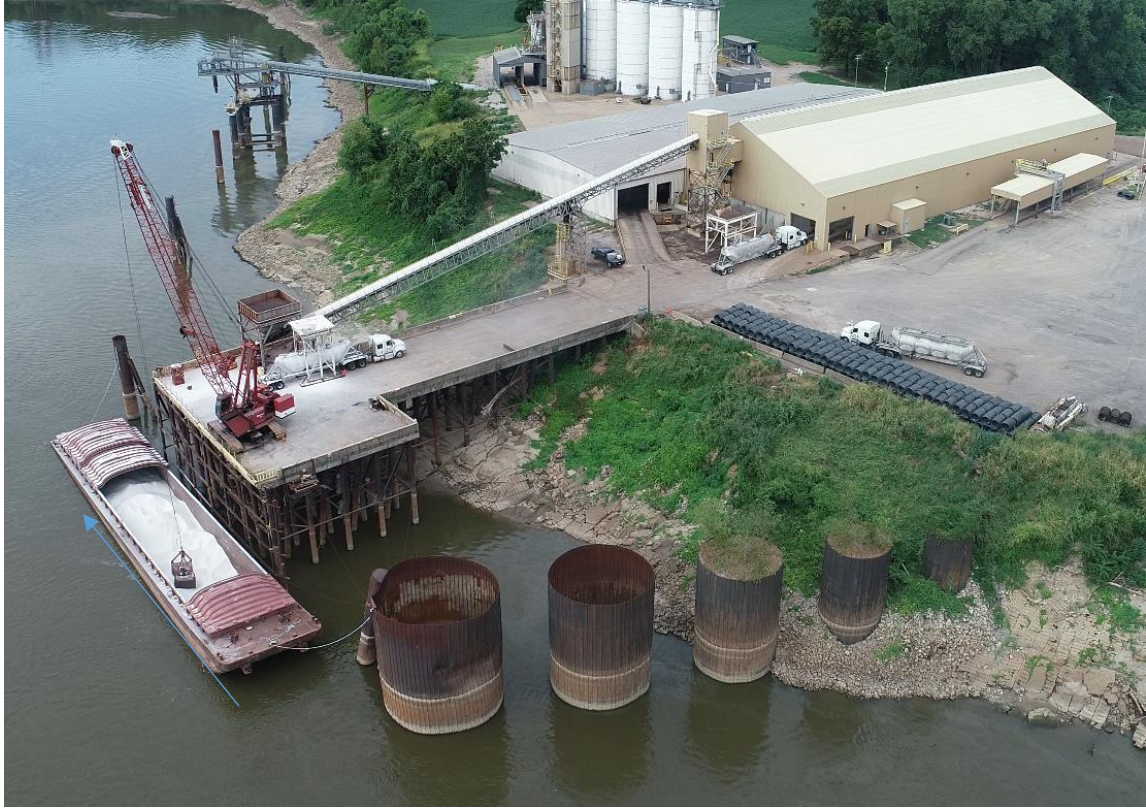
Figure 1. Dock configuration at low water with barge docked (flow direction arrows in blue)
