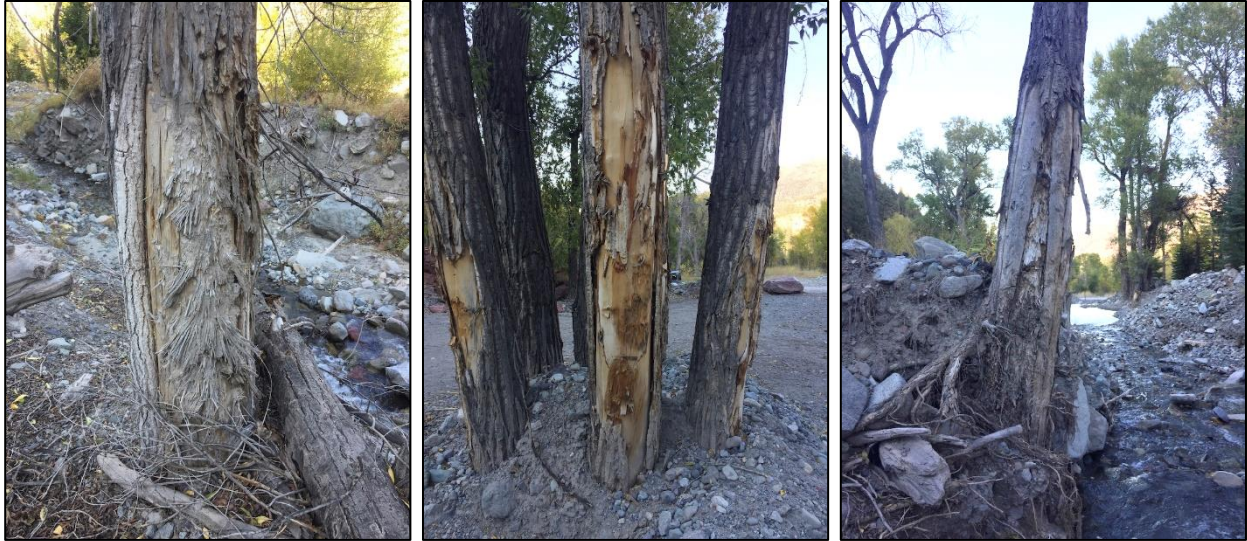
Figure 1. Observed scour marks on trees from past debris flows
