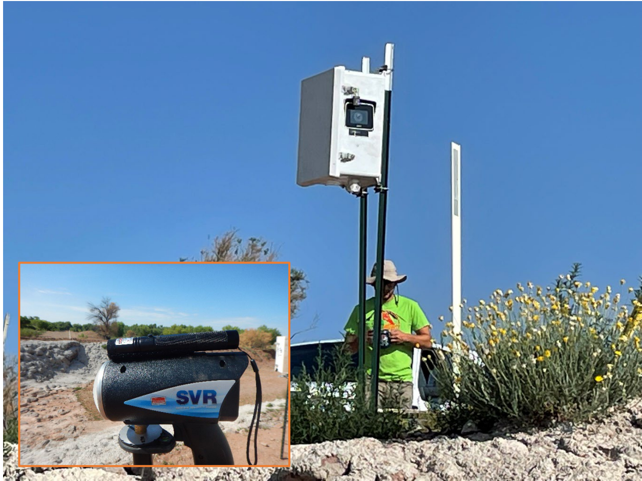
Figure 2. Instruments added to site for surface velocity measurements: mounted LSPIV camera in protective housing; Inset is of handheld radar
