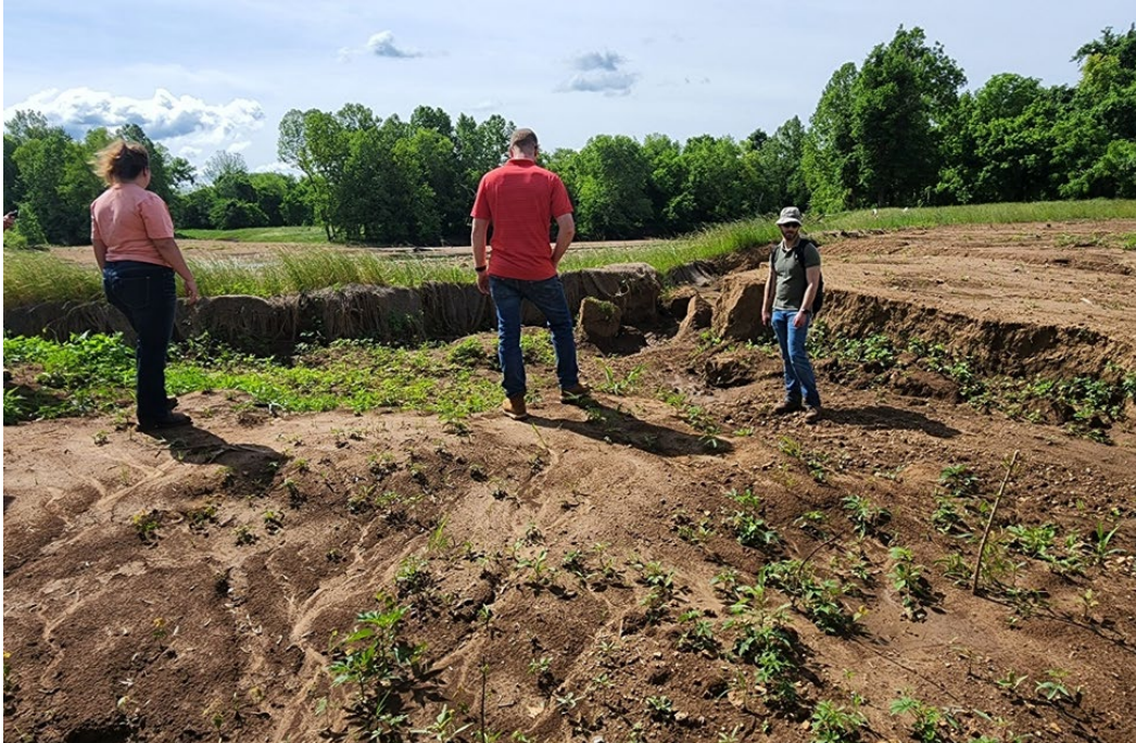
Figure 25. Bank 1 monitoring - scour at crest of shaped bank. Bluff behind photographer; floodplain to the right; Big River flowing from left.
