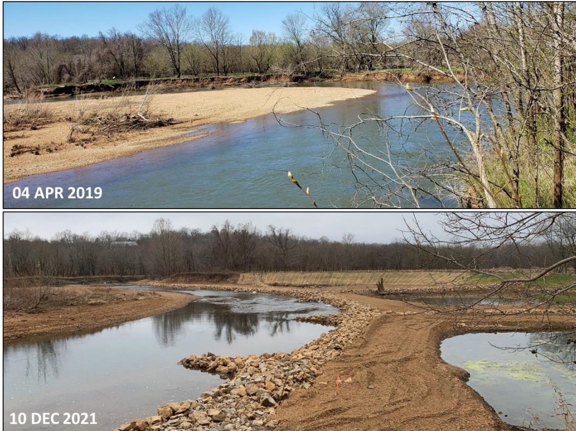
Figure 21. Bank 1 pre- and post-construction. Facing downstream.
