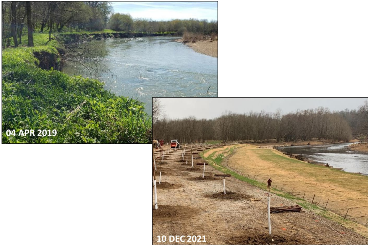
Figure 1. Bank 3 pre- and post-construction. Facing upstream.
