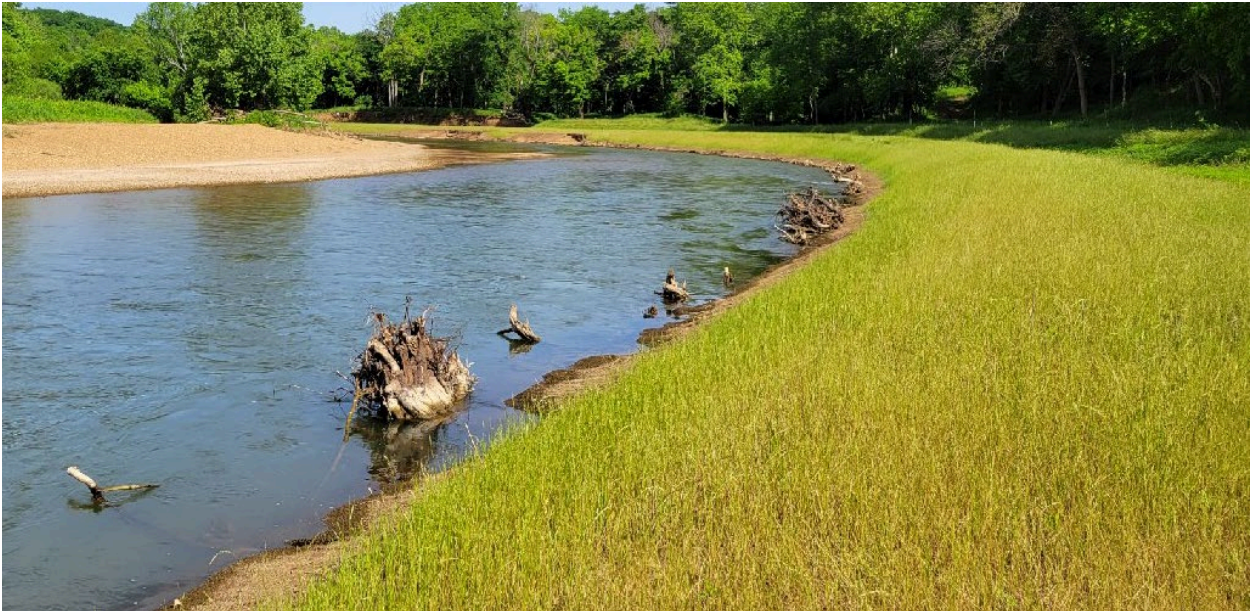
Figure 26. Bank 3 monitoring - performing well overall. Facing downstream.
