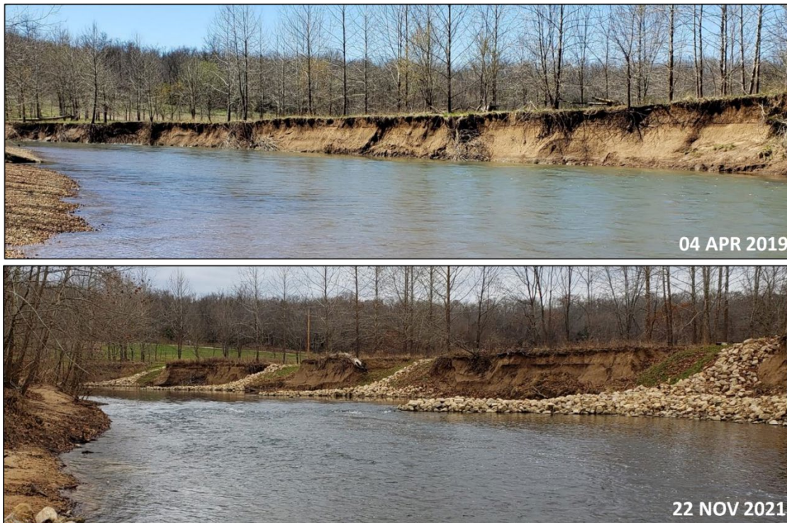
Figure 23. Bank 2 pre- and post-construction. Facing upstream.
