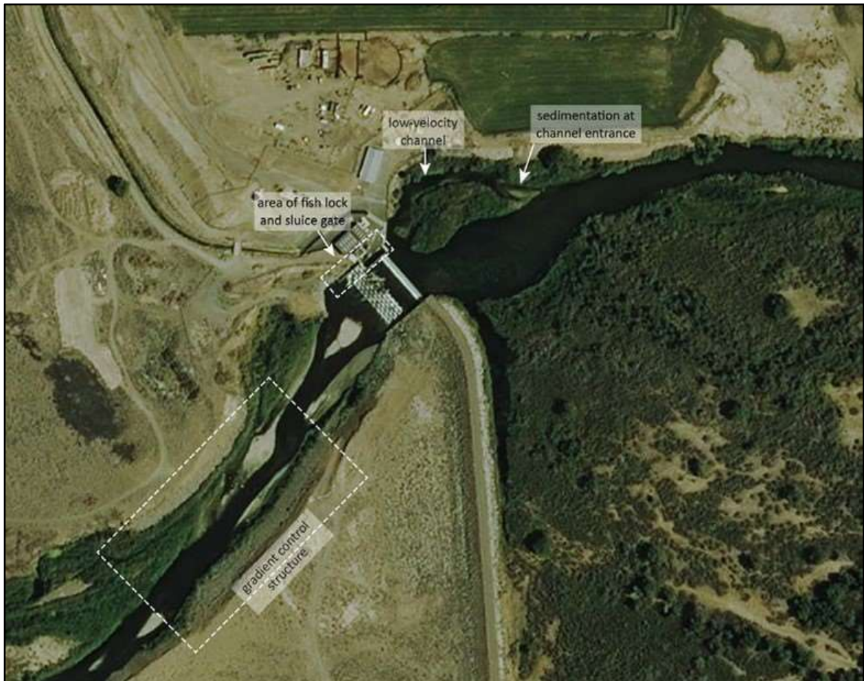
Planview of Marble Bluff Dam facility near Nixon, NV about Five miles Upstream of Pyramid Lake.
